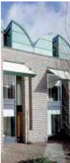
Mews houses, Dublin. Architect: de Blacam and Meagher. Copper Contractor: Miskin Services.
