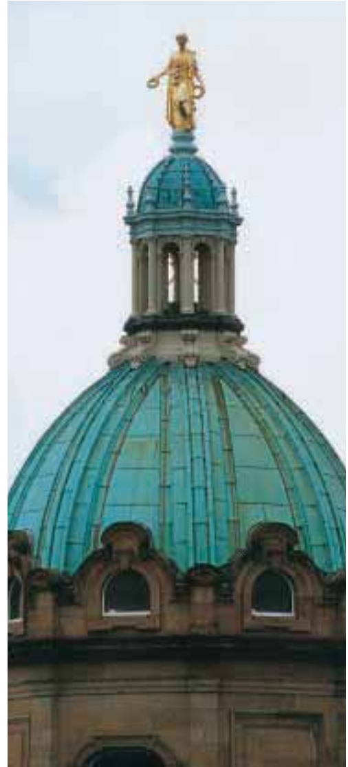
Renovation of top dome, Bank of Scotland HQ, Edinburgh. Roofing Contractor: D. Blake & Co.
