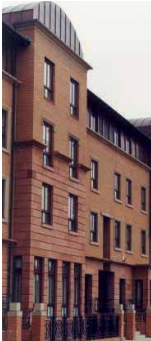
The Crown Street Regeneration Project, Gorbals, Glasgow. Architect: Hypostyle. Roofing Contractor: A & J Roofing Specialists.
