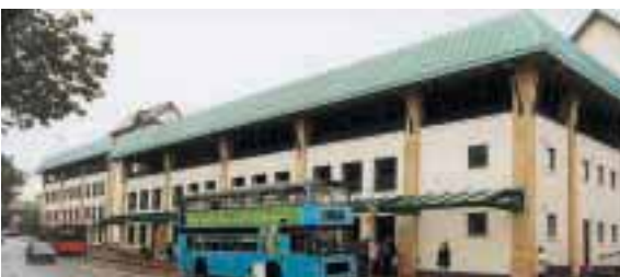
Multi-storey car park, Caernarfon. Designers: Adams Consulting Engineers. Roofing Contractor: Varla (UK).
