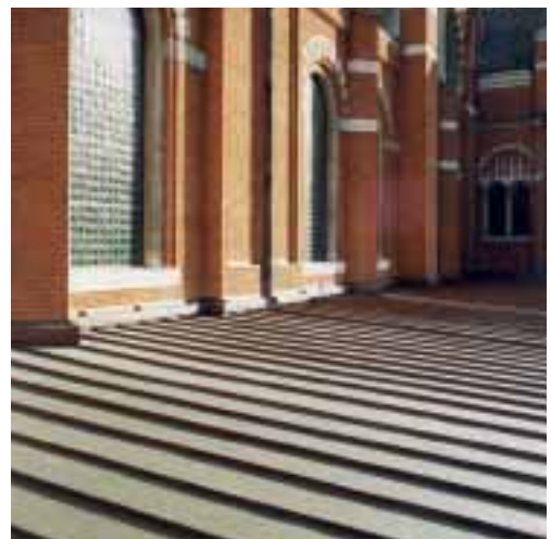
Chapel Roof at Westminster RC Cathedral, London. Architect: John Phillips. Roofing Contractor: L S Smerald.
