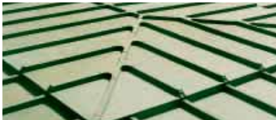
Traditional batten roll method.
