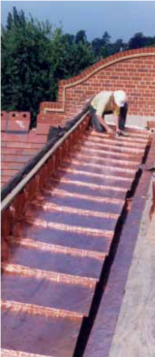
Copper roof installation at Linacre College, Oxford.
