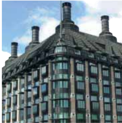
Copper alloy cladding at Portcullis House, London. Architect: Michael Hopkins and Partners. Roofing/Façade Contractors: Watson Steel/Seele Alvis Fenestration.
