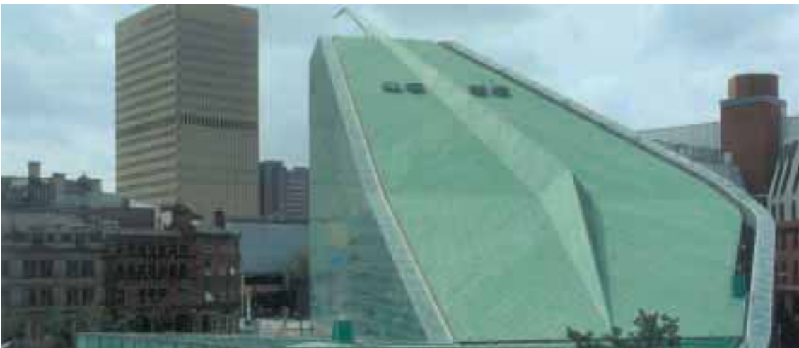
Urbis, Manchester. Architect: Ian Simpson Architects. Copper Contractor: Varla (UK).
