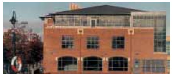
Profiled sheet roofing on commercial offices, Belfast. Architect: Knox & Markwell. Roofing Contractor: Edgeline Contracts.
