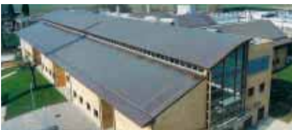
Unilever Research Laboratory, Colworth House, Sharnbrook. Architect: Sheppard Robson. Roofing Contractor: Kelsey Roofing.
