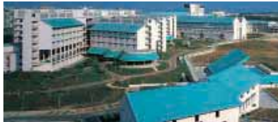
Temasek Polytechnic, Singapore. Architect: Stirling Wilford.
