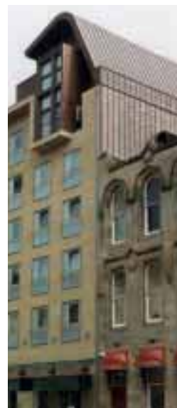
Brunswick Hotel, Glasgow. Architect: Elder & Cannon. Roofing Contractor: A & J Roofing Specialists.
