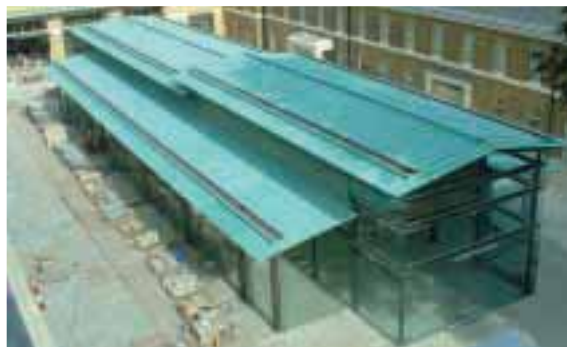
Duke of York's Headquarters, London. Architect: London Bloc Architects. Copper Contractor: T+P Lead Roofing.
