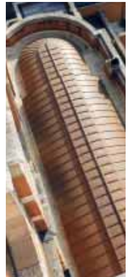
Westminster R C Cathedral, London. Architect: John Phillips. Roofing Contractor: L S Smerald.
