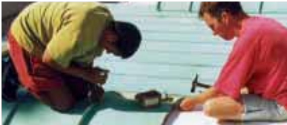
Installation of pre-formed curved trays.
