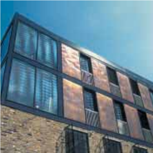
2 Newhams Row, London. Architect: Glas Architects and Designers. Copper Contractor: Metalex.
