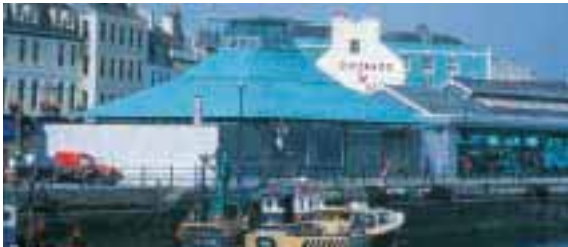
Dartington Glass Works, Plymouth. Architect: Form Design Group. Roofing Contractor: J E Gibbins & Sons.
