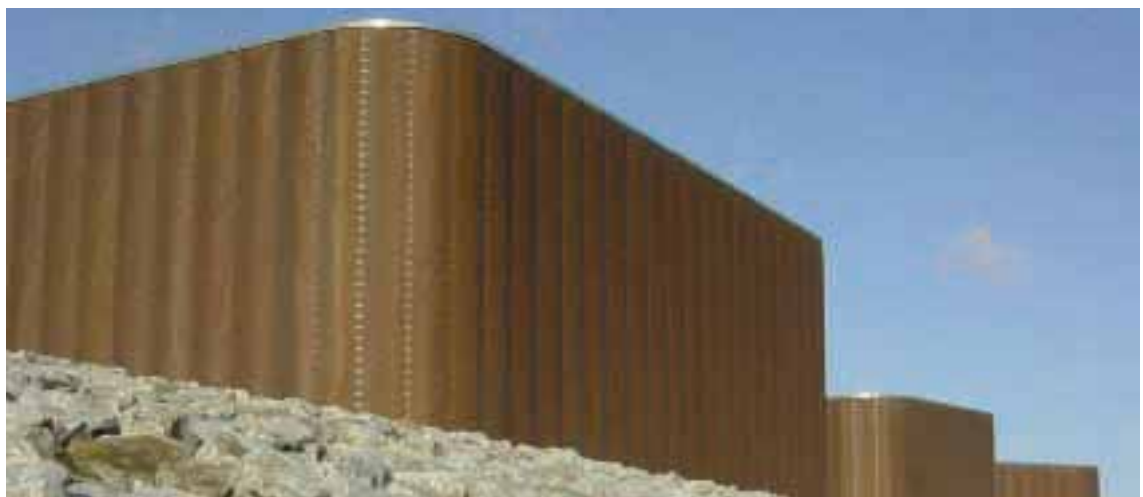
Copper alloy mesh cladding at Plymouth Theatre Royal Production Centre. Architect: Ian Ritchie Architects. Copper Contractors: Lockerwire Weavers/Rubb TM.
