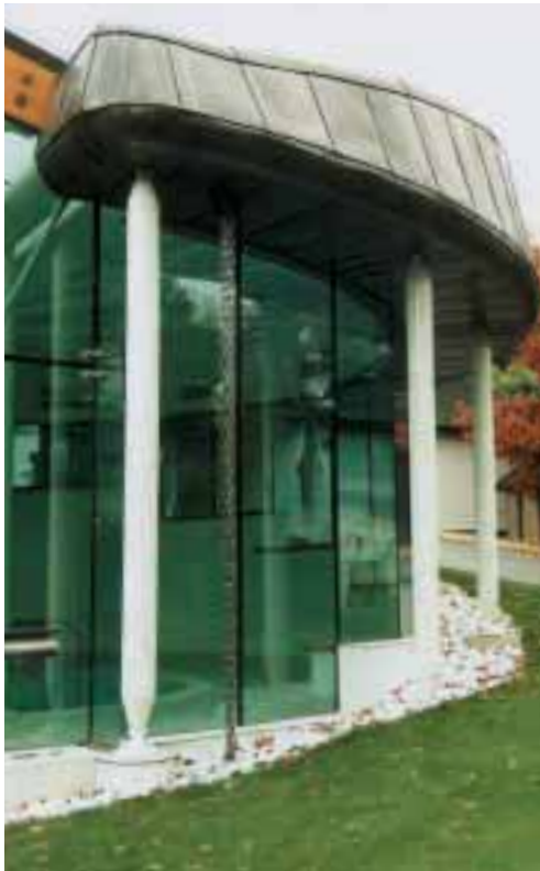
Private house swimming pool annexe, Berkshire. Architect: Trinéire Designs. Roofing Contractor: Cotswold Metal Roofing.
