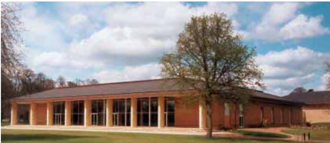
The Masonic School, Rickmansworth. Architect: Walton Smart Associates.
