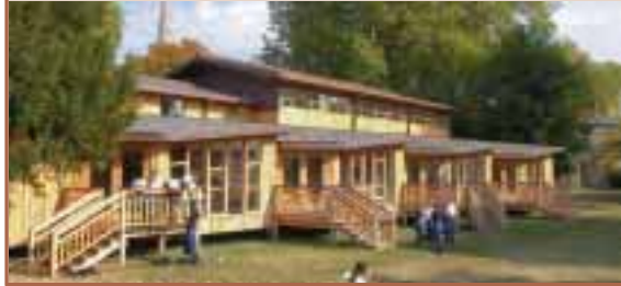
Architect: Keith Harnden.
