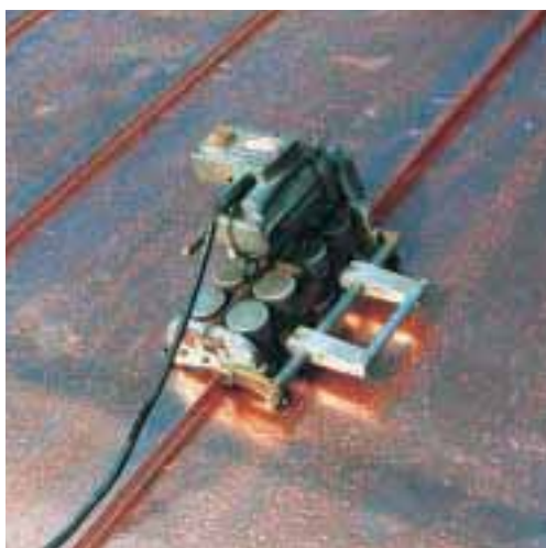
Mechanised seaming, Long Strip system.
