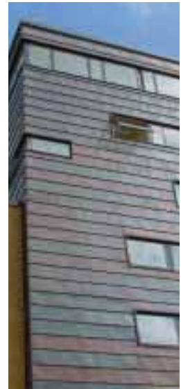
University College London. Architect: Feilden Clegg Bradley Architects. Copper Contractor: NDM.
