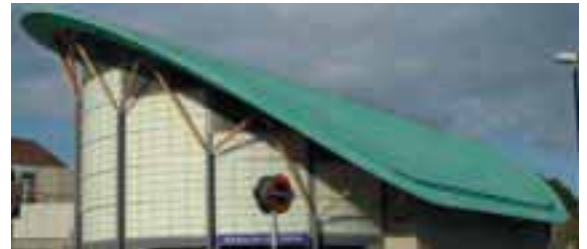
Hounslow East Station, London. Architect: Acanthus Lawrence & Wrightson. Copper Contractor: Brodericks.
